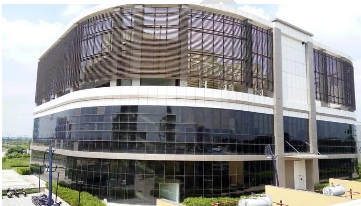
District Cooling Plant at GIFT City
